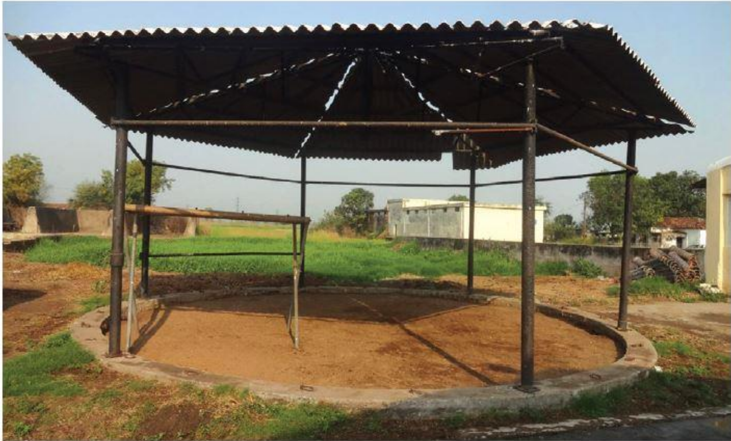
Casting pit filled with sand as bedding
